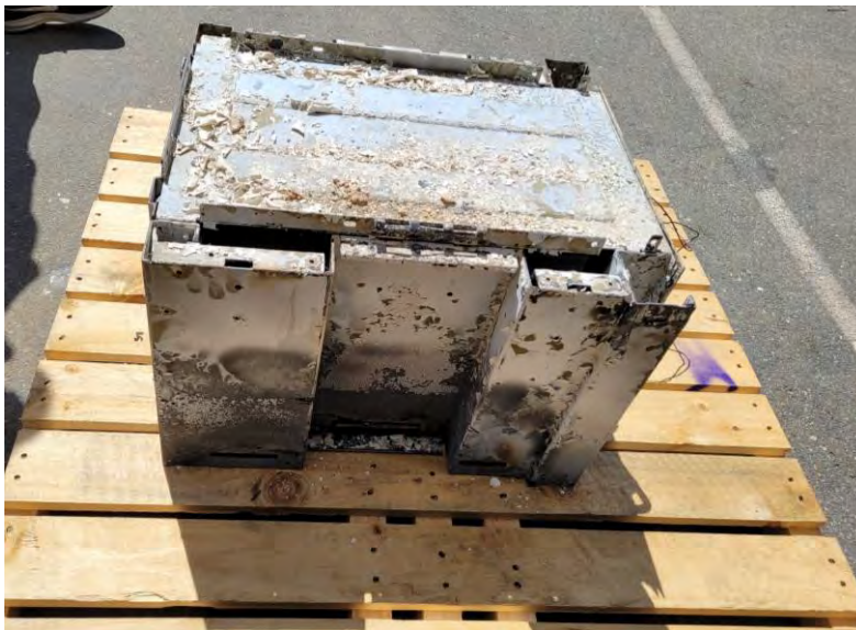
Picture 8 – Unit BBU – Unit After Exposure at 950°C
