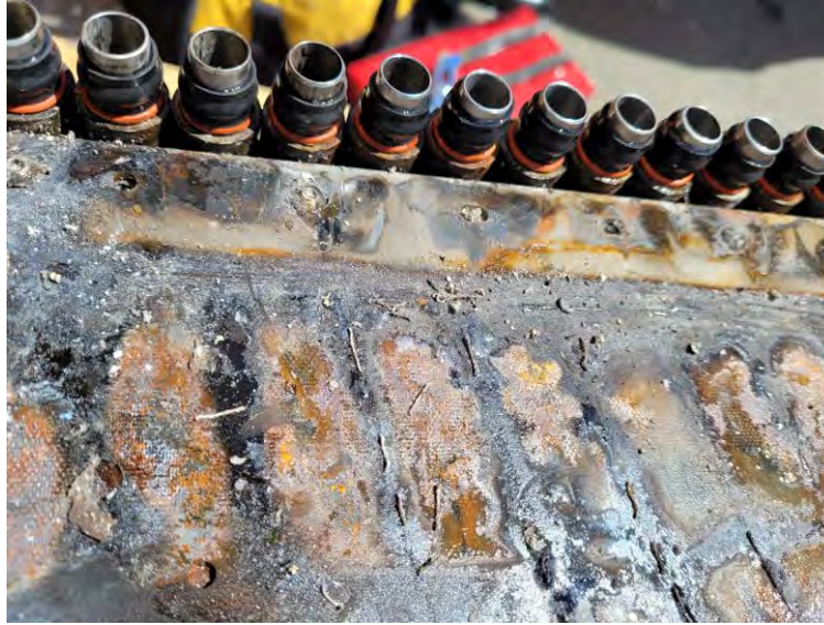
Picture 15 – Unit BBU – Unit After Exposure at 950°C – Water Coolant System Caps Removed – View of Gaskets
